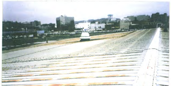
"A Metal Roof Before Retrofit"
