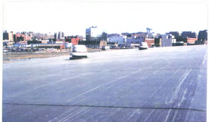
Metal Roof Retrofitted with EPDM
