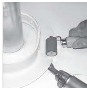
3. Heat weld vertical &amp; horizontal seams first
