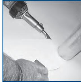
1. Overlay cut in TPO Membrane
