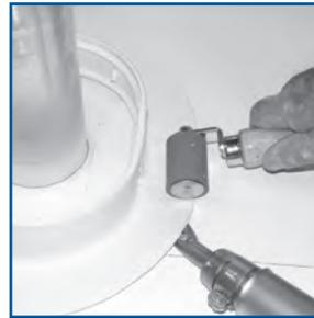
3. Heat weld vertical &amp; horizontal seams first
